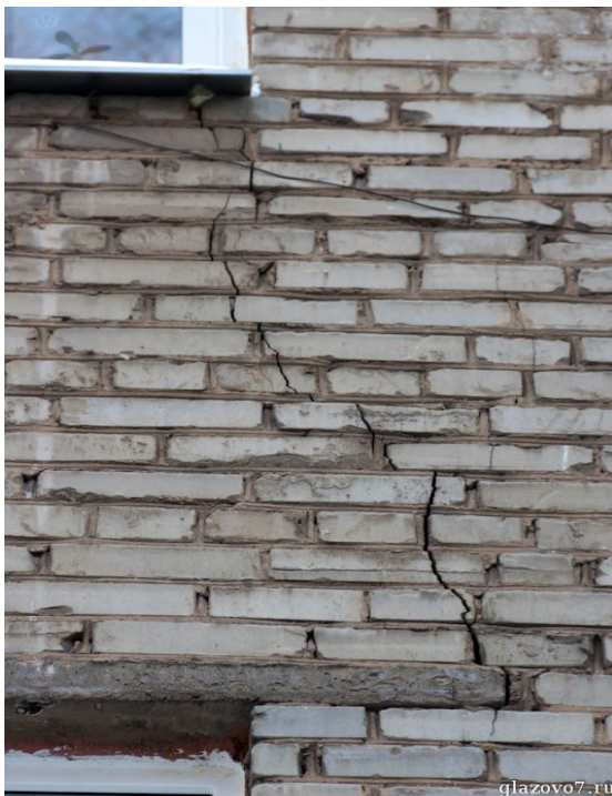
Figure 2. Cracks under the windows
