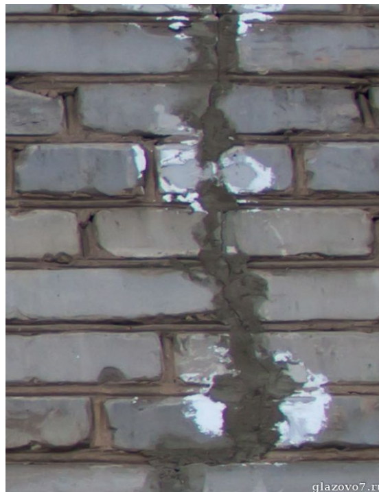
Figure 2. Cracks under the windows
