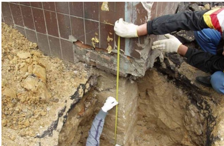
Figure 3. Inspection of structures of foundation elements
